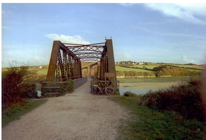
Iron Bridge Padstow
